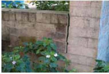
Photo No 90 (SE retaining wall)
