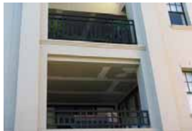
Photo No 79 (repaired balcony ceilings below Unit 301)
