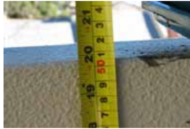
Photo No 80A (Unit 301 NW balcony balustrade)
