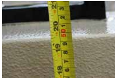
Photo No 63a (unit 302 West balcony balustrade)
