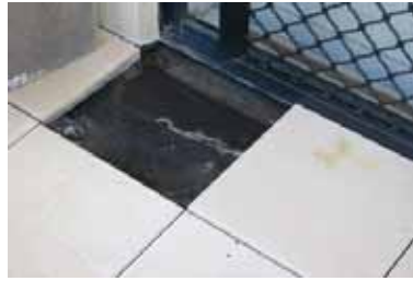
Photo No 78 (Unit 301 west balcony)
