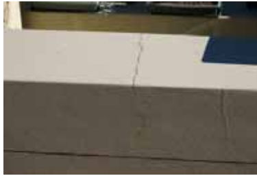
Photo No 82 (Penthouse western balcony balustrade)
