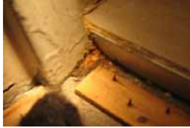
Photo No 73 (unit 302 bathroom entry door)
