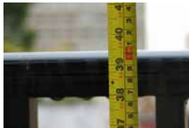
Photo No 64 (unit 302 West balcony balustrade)
