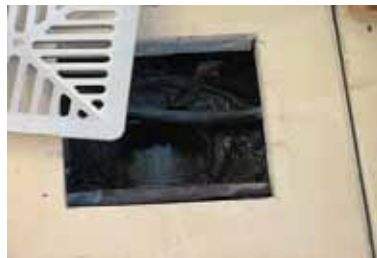
Photo No 78A (Unit 301 west balcony)
