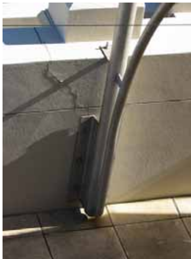
Photo No 83 (Penthouse western balcony balustrade)
