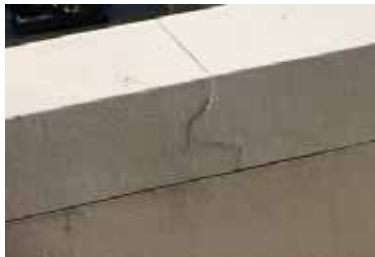
Photo No 82A (Penthouse western balcony balustrade)
