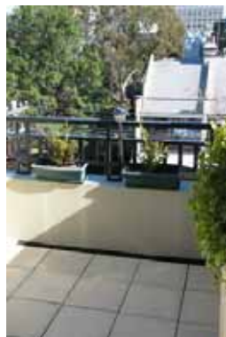
Photo No 80 (Unit 301 west balcony balustrade)
